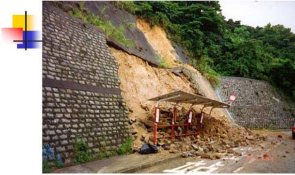
Near ground surface, engineered structures become unstable in response to extreme changes in moisture flux boundary conditions
