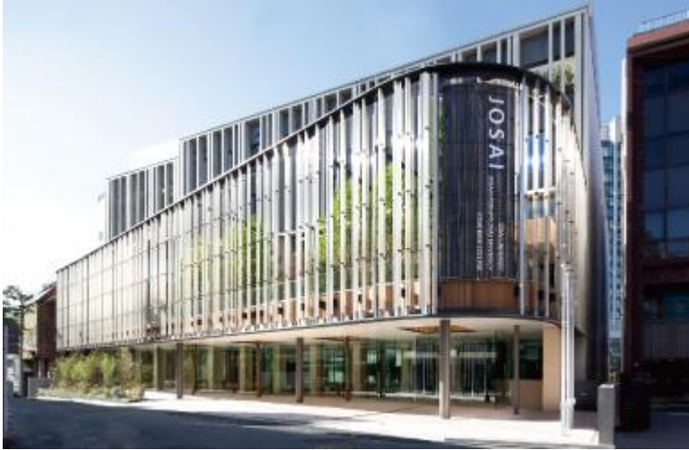
JIU Campus Building No. 3
