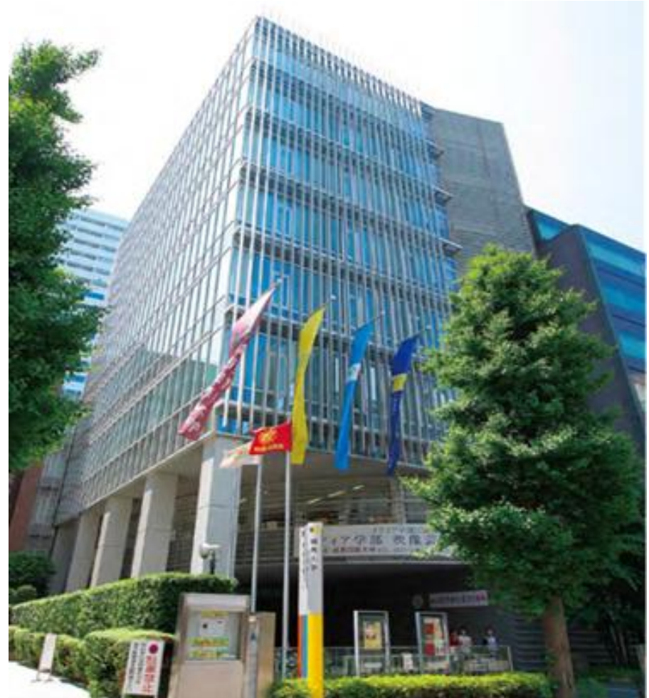
JIU Campus Building No.1
